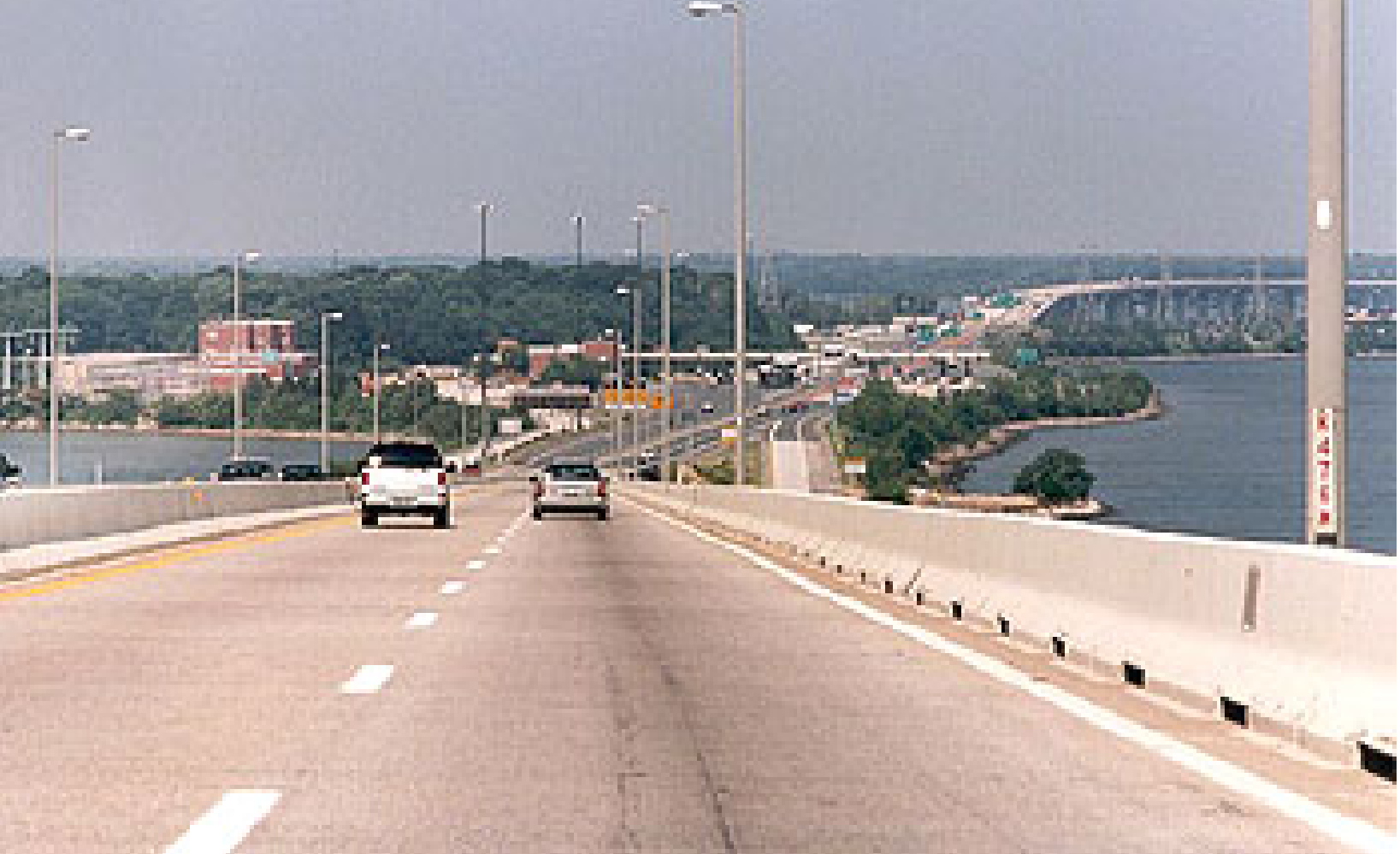
Above, on the Key Bridge, northbound, just north of the continuous truss span, looking toward the toll plaza, and the Bear Creek Bridge (Sparrows Point Viaduct) in the distance. Photo taken July 5, 1999, the Monday that was the holiday for Independence Day in 1999; at about 3:00 PM, near the end of a holiday weekend which is one of the highest interstate travel days of the year. The 3.5-mile-long widening project to widen the 2-lane Sparrows Point section was still under construction. As you can see, the eastern portion of the I-695 Baltimore Beltway has capacity to spare. This should provide an effective I-95 bypass for many years into the future. Click the photo for large image (112K).
