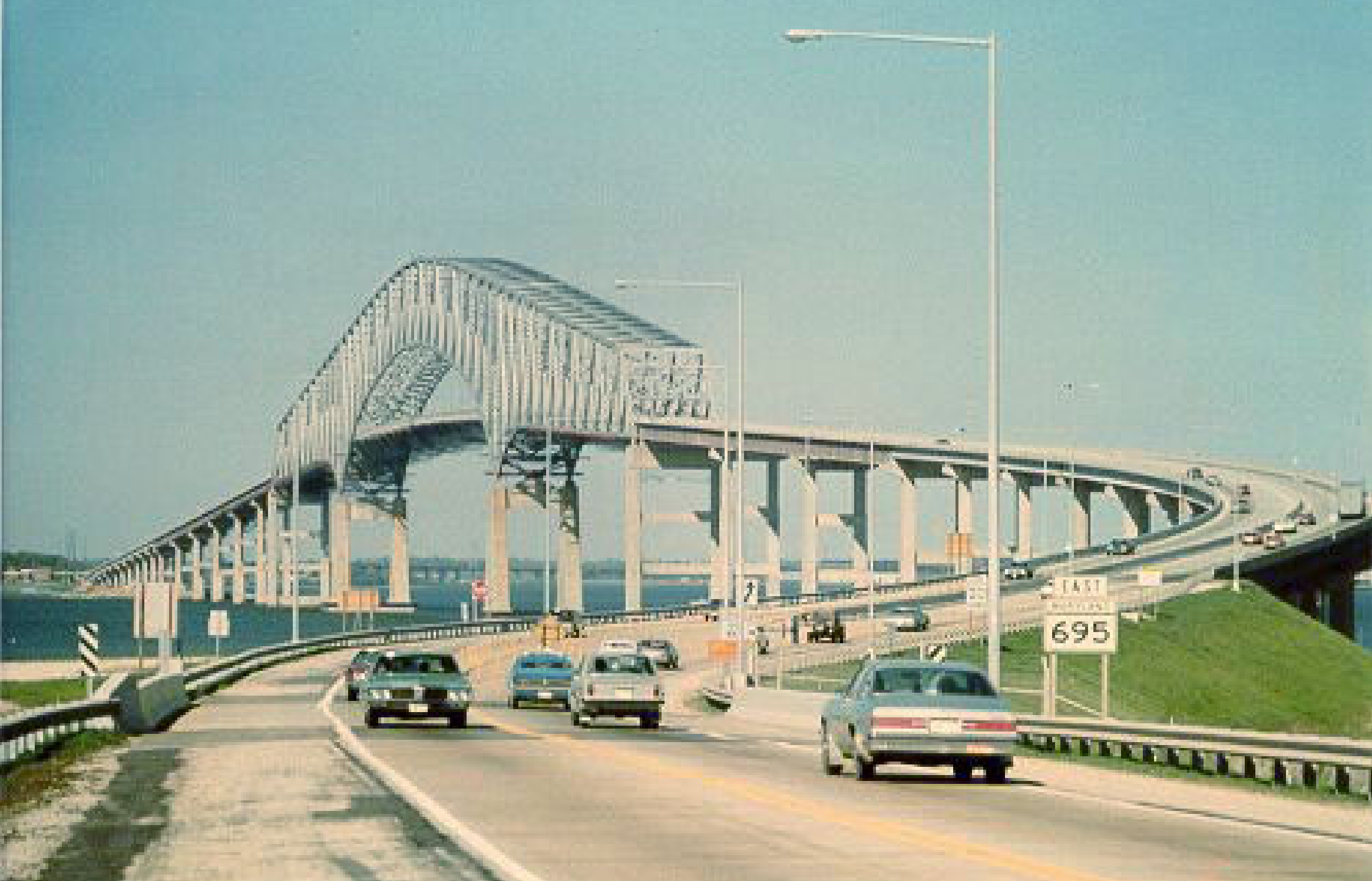
Above, Key Bridge, looking north, taken in April 1978. The south approach was two lanes, and was widened to four lanes by 1981. Note that the road was MD-695 originally. Notice the safety nets hanging under main span, as the original painting was finishing up.
