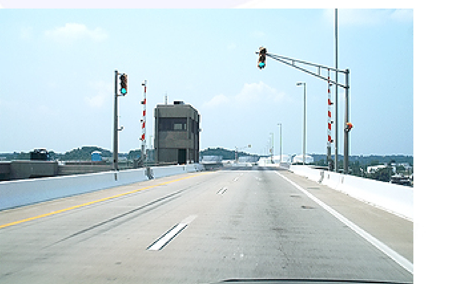
Above, eastbound Curtis Creek Bridge on I-695, on the Outer Harbor Crossing, three miles west of the Key Bridge. This crossing is comprised of twin bridges, each with two lanes, and each with a bascule drawspan with 60 feet of vertical navigational clearance when closed. Click the photo for large image (178K). Photo offered to this website, August 2002, by Rush Wickes of Blacksburg, Virginia.
